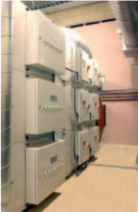
Six ESP and Three UV-C modules installed as an integrated system.
